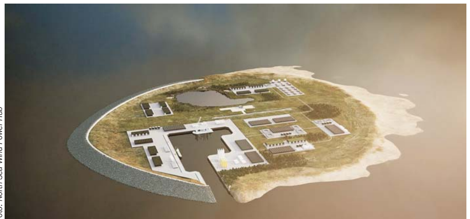
Foto: North Sea Wind Power Hub
