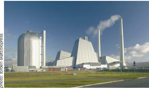
The Avedøre plant, which is to use 300,000 tonnes of wood pellets annually.
