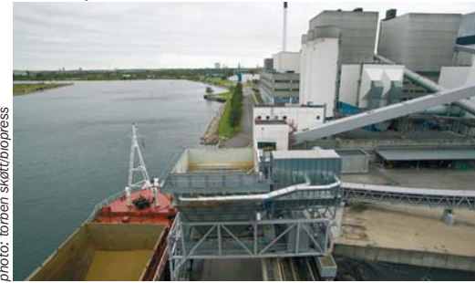
The coaster "Grethe" unloading straw pellets for the Amager plant.
