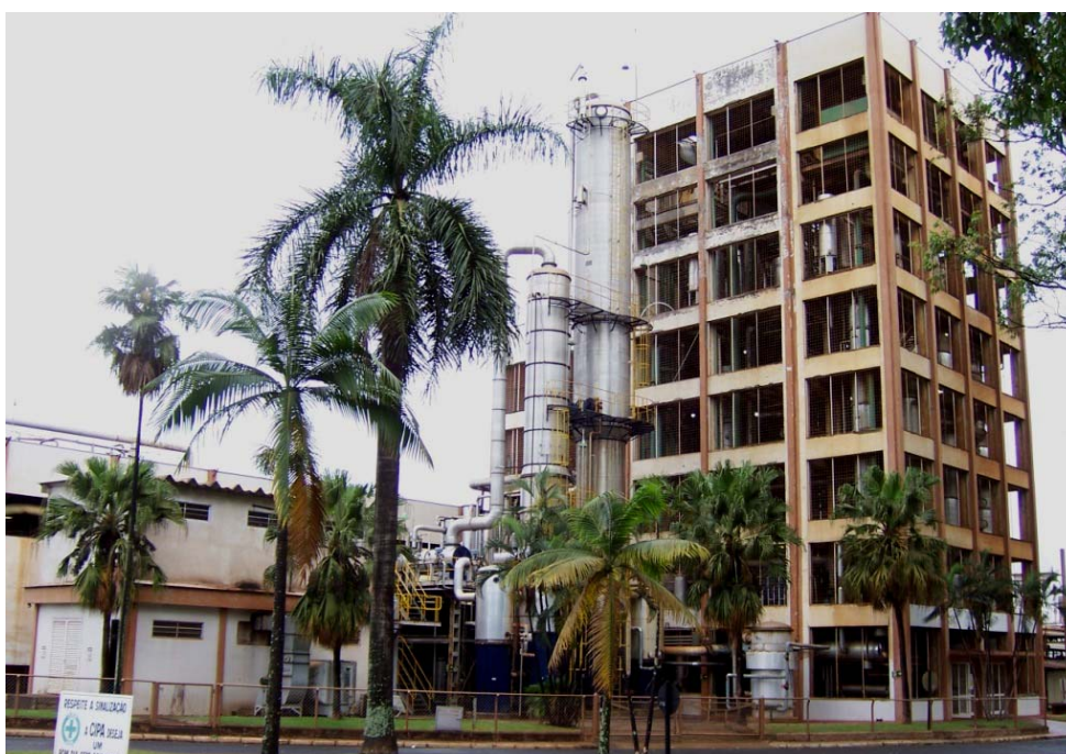
Figure 19: Distillery for bioethanol production from sugarcane in Brazil.
